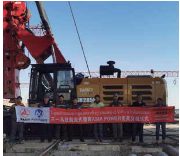
SR285R at Uzbekistan railway project
