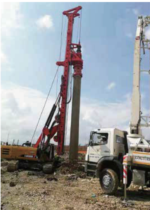
SR285R Casing construction method works in Turkey
